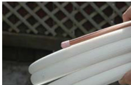
Figure 6.3 Cover pipe ends
