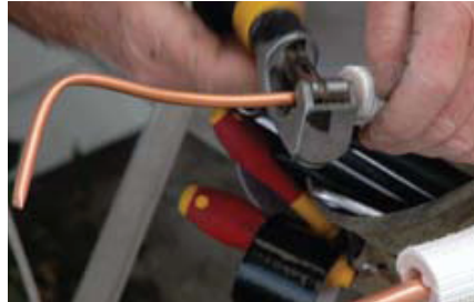
Figure 6.5 Cut pipe with tube cutters
