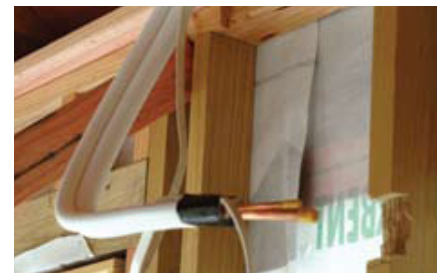
Figure 6.19 Notch the top plate and studs (B)
