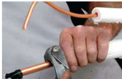
Figure 6.2 Pipe opening facing down when cutting
