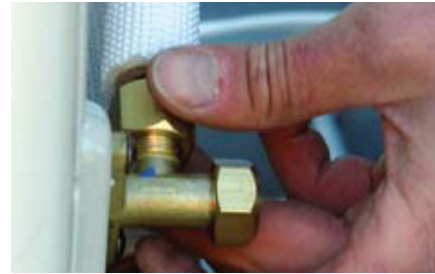
Figure 6.14 Connect the pipes (B)
