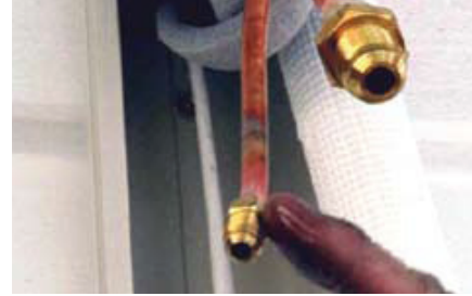
Figure 6.12 Apply oil to the back of the flared pipe and the flare joint
