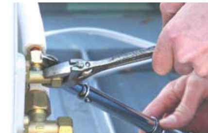
Figure 6.15 Tighten connection (A)
