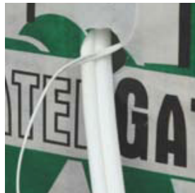
Figure 6.24 Feed pipe/cables through building wrap
