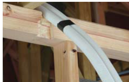
Figure 6.18 Notch the top plate and studs (A)
