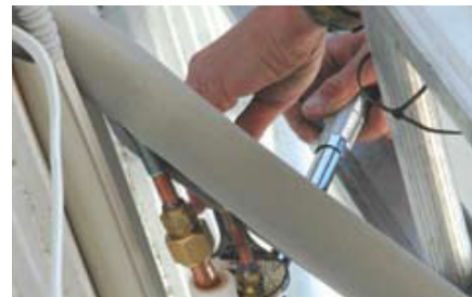
Figure 6.16 Tighten connection (B)
