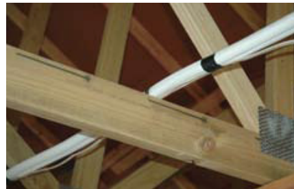
Figure 6.17 Run pipe/cable across truss chord/ceiling joist
