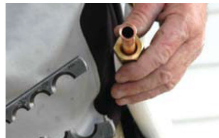
Figure 6.10 Flare the end of the tube (C)
