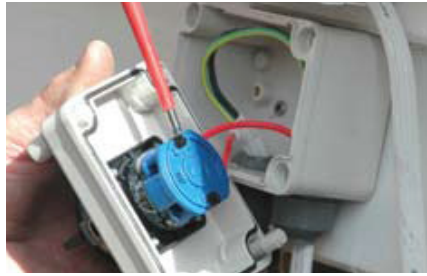
Figure 9.4 Install lockable isolating switch (C)
