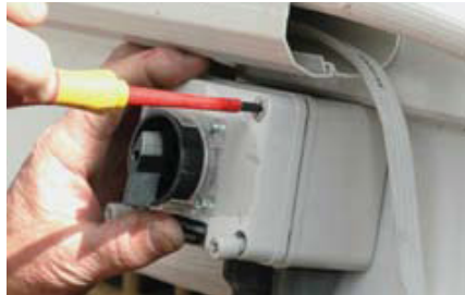
Figure 9.4 Install lockable isolating switch (C)
