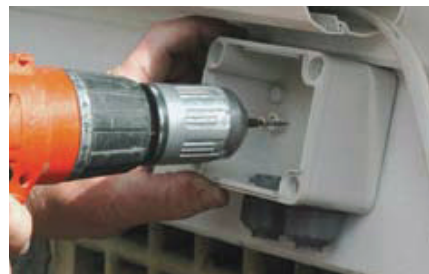
Figure 9.2 Install lockable isolating switch (A)
