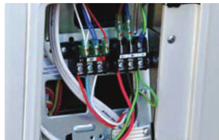
Figure 9.1 Connect power supply cable to terminal block
