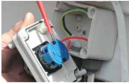
Figure 9.4 Install lockable isolating switch (C)
