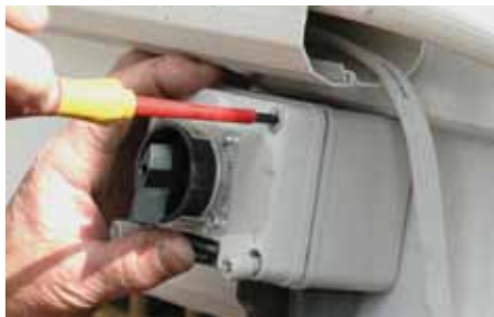
Figure 9.4 Install lockable isolating switch (C)
