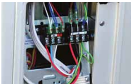
Figure 9.1 Connect power supply cable to terminal block
