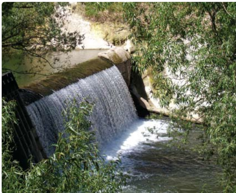
Using abandoned or decommissioned hydro infrastructure may be a cost-effective basis for a hydro scheme.
