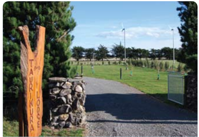
The lodge has two grid-connected Skystream wind turbines.
