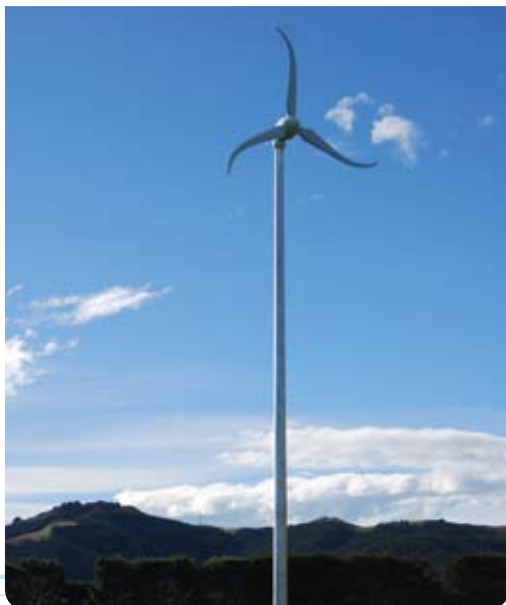
The turbines are on 10 m high poles.
